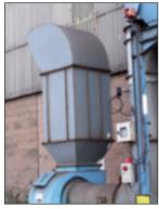
Networked Electrodynamic<sup>®</sup> Sensor used to remotely pinpoint bag row failure on a moulding sand plant
